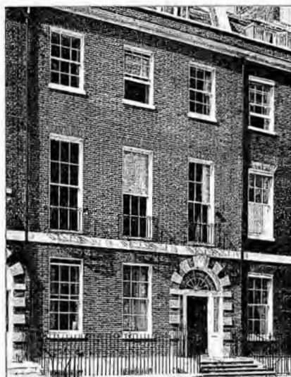
Fig.5 Several houses in Bedford Square, such as No.23 here, have deliberately blackened stock brickwork, pointed in contrasting white mortar. Although built between c.1775 and 1782, this treatment may only date from the late nineteenth century. (RCHME, Crown copyright)
