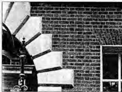
Fig.3 Detail of the fine brickwork on No.44 Berkeley Square.
